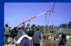
Installation Process, carrying wind turbine
