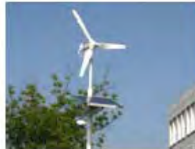
Solar street lighting (combined a solar panel, wind turbine )
