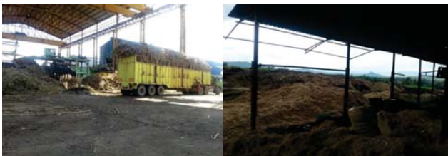
Figure 1: Bagasse production and storage in the factories
