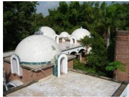
Figure 21. Roof top view
