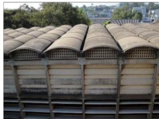
Figure 17. Ventilated roof top view
