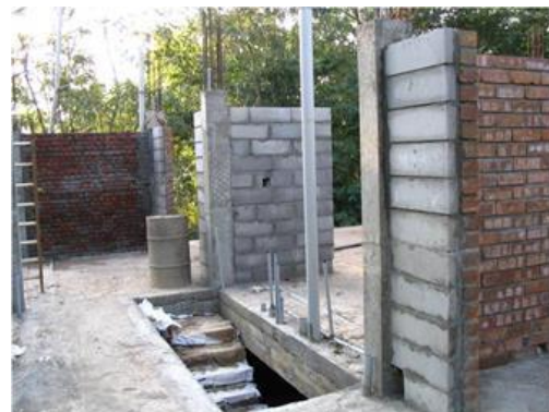
Figure 13. Composite wall (construction) With ACC and Earth blocks
