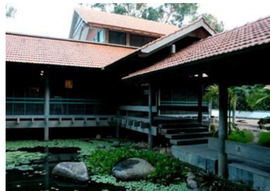
Figure 29, Dining hall protruding into pond, Afsanah guest house
